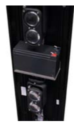
MANA BH NEW CABLE PIT BATTERY SUPPORT
